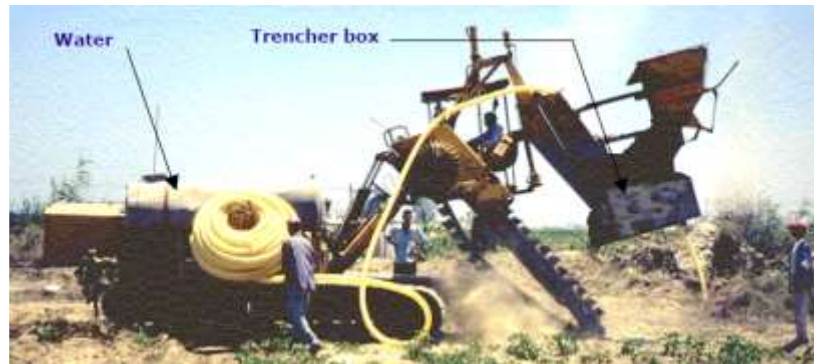
Figure 2. Spraying the trencher box with water to reduce friction with the soil
